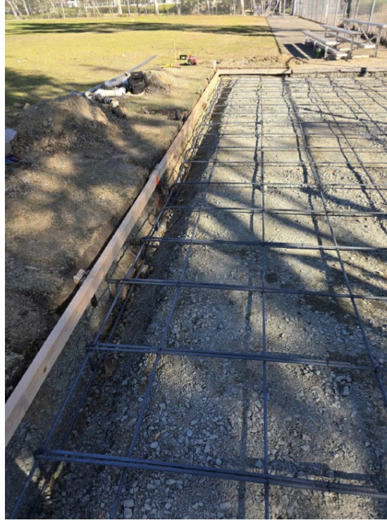
Rebar Placed at Practice Field
