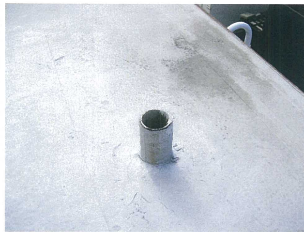
PHOTO # 2 Vent Pipe
