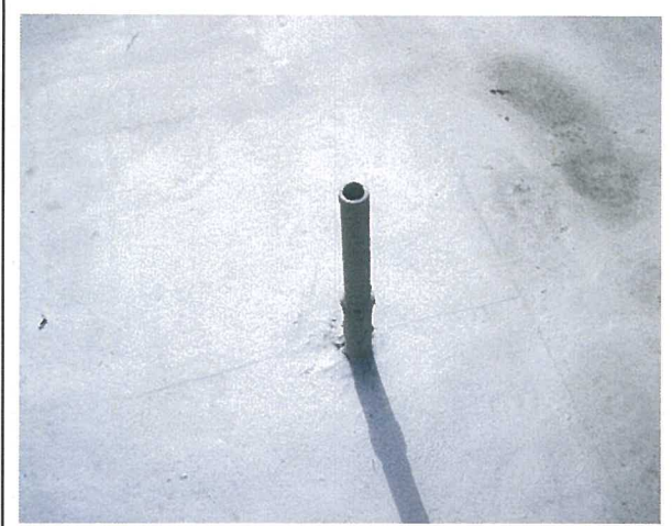
PHOTO # 3 Vent Pipe
