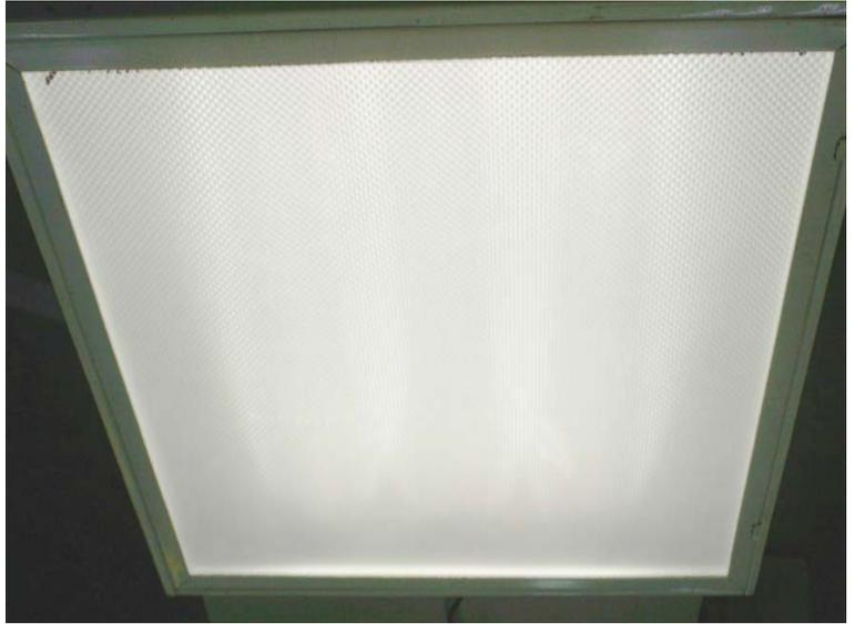
S2-3-28W-35K STRIPIT KIT™ installed in a Lithonia SP8 2X2 Prismatic Troffer. Even with only three strips installed, because of the deep location and the diffusers the ‘fill’ of the A12 lens is very uniform with none of the ‘banding’ effect complained about with most LED retrofit systems.
