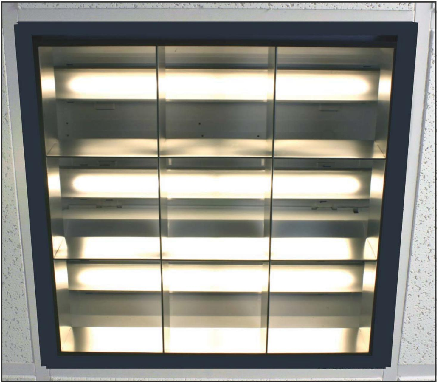
A STRIPIT KIT™ retrofit in a 2X2 parabolic troffer previously populated with fluorescent U-tubes
