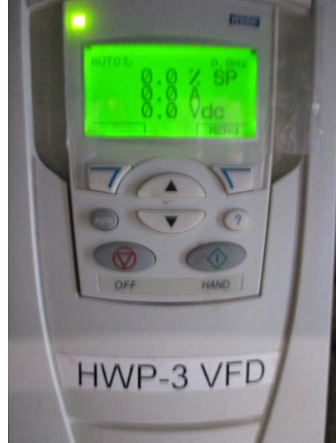
Figure 30 – HW Pump VFD
