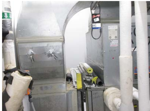
Figure 18 – Floor Mounted Fan Coil Unit
