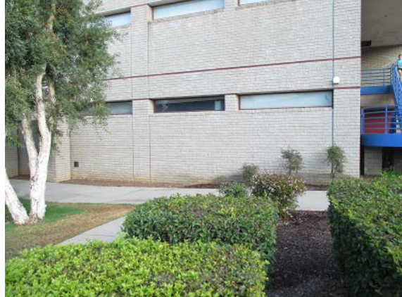
Figure 16 – Building Exterior and Windows 1
