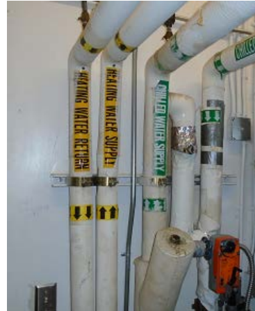
Figure 10 – 4-Pipe Configuration
