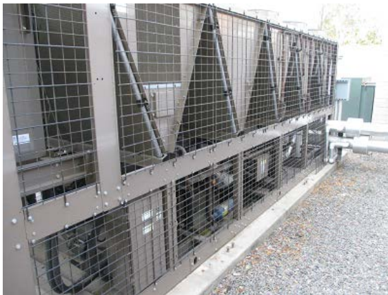
Figure 3 – Screw Chiller
