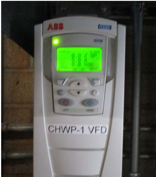
Figure 29 – CHW Pump VFD
