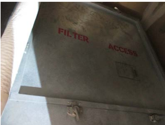
Figure 19 – Fan Coil Filter Access
