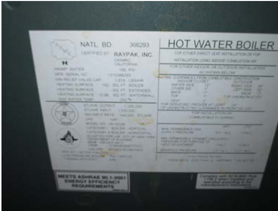
Figure 27 – Boiler Nameplate
