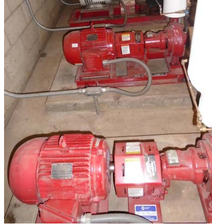
Figure 6 – Heating Hot Water Pumps
