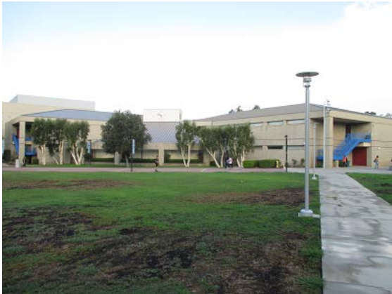
Figure 15 – RSCCD Building D
