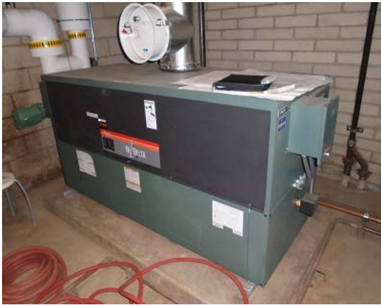
Figure 5 – Heating Hot Water Boiler
