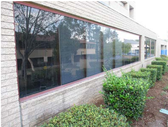
Figure 17 – Building Exterior and Windows 2
