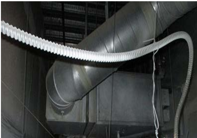
Figure 9 – Fan Coil Unit on Hangers
