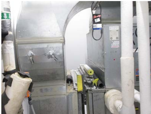
Figure 7 – Floor Mounted Fan Coil Unit
