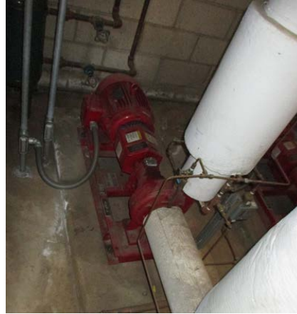
Figure 28 – Hot Water Pumps
