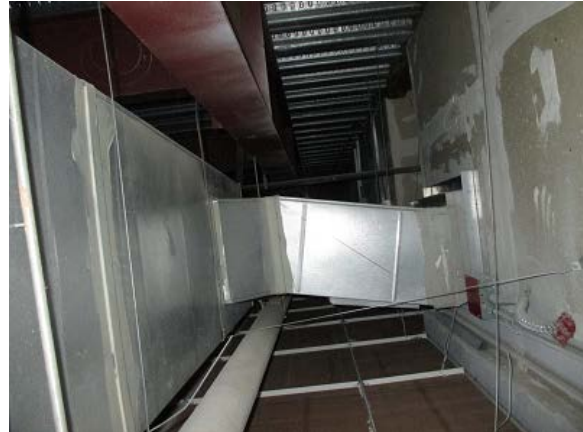
Figure 8 – Ceiling Fan Coil Unit
