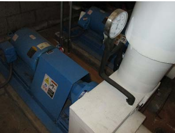
Figure 25 – Chilled Water Pumps
