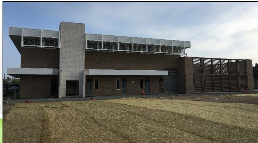
New Central Plant
