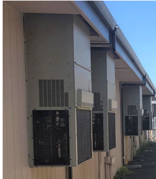
Newly installed upgraded HVAC Units
